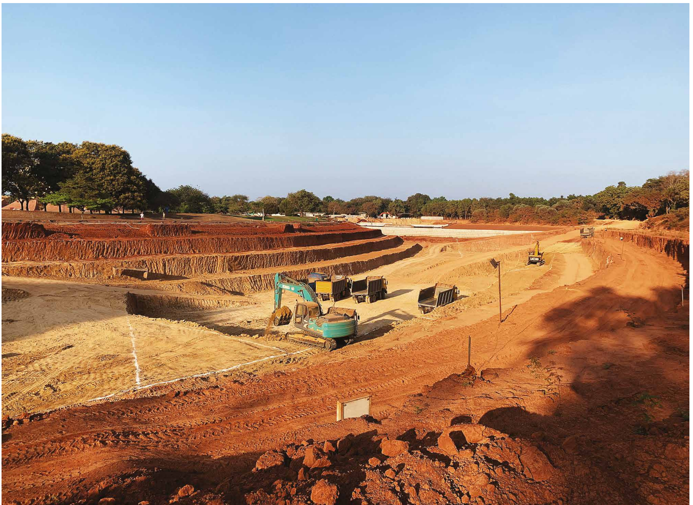
Excavation underway for Lake section 2
